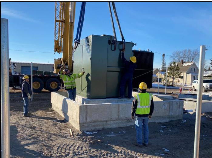
Crews are setting the 37,000 lb, 7.5m VA transformer for a new substation located near 10th St S and 1st Ave.
