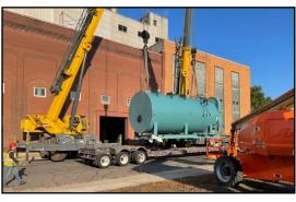
With the completion of the Northside steam zone conversion last November our larger boilers could not be operated in the summer at a low enough level to stay in compliance. Because this boiler has the ability to modulate, meaning it can turn off and on based on the outlet steam pressure, it can easily operate at the lower system pressures. In addition, this boiler, operating at full capacity, is capable of carrying the steam district on its own on the coldest of winter days.
